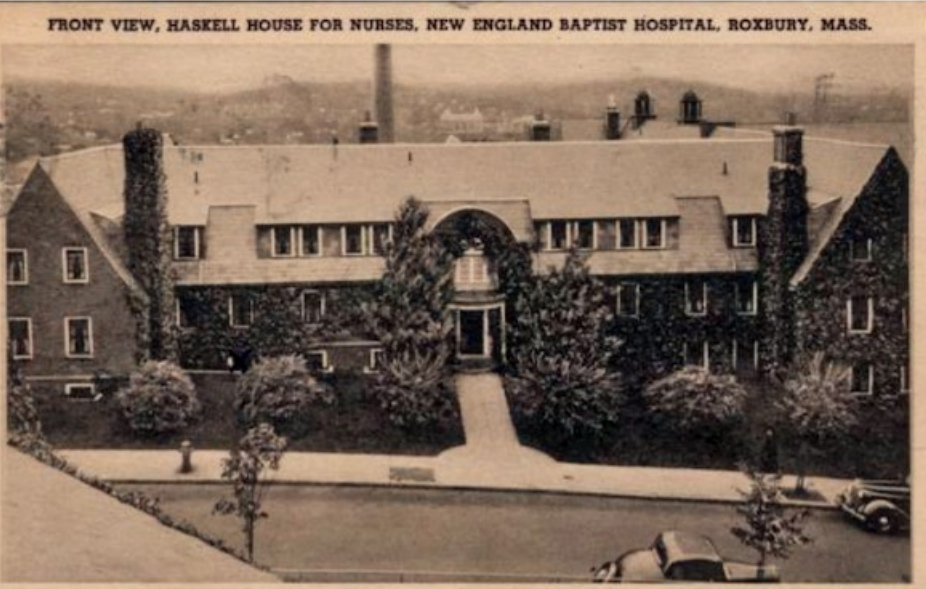
A historic postcard from the 1930s shows Haskell House in use as the nurses dorm at New England Baptist Hospital. The BPDA board swept aside neighbors’ concerns in July to approve the building’s conversion to apartment units.
