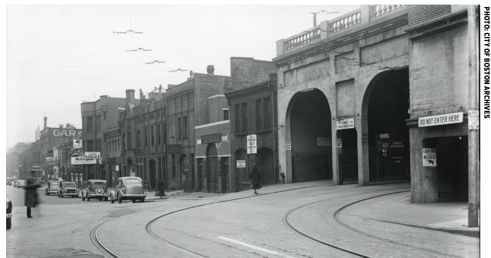
Mass Ave Streetcar Station on the Newbury Street side in the 1930s.
