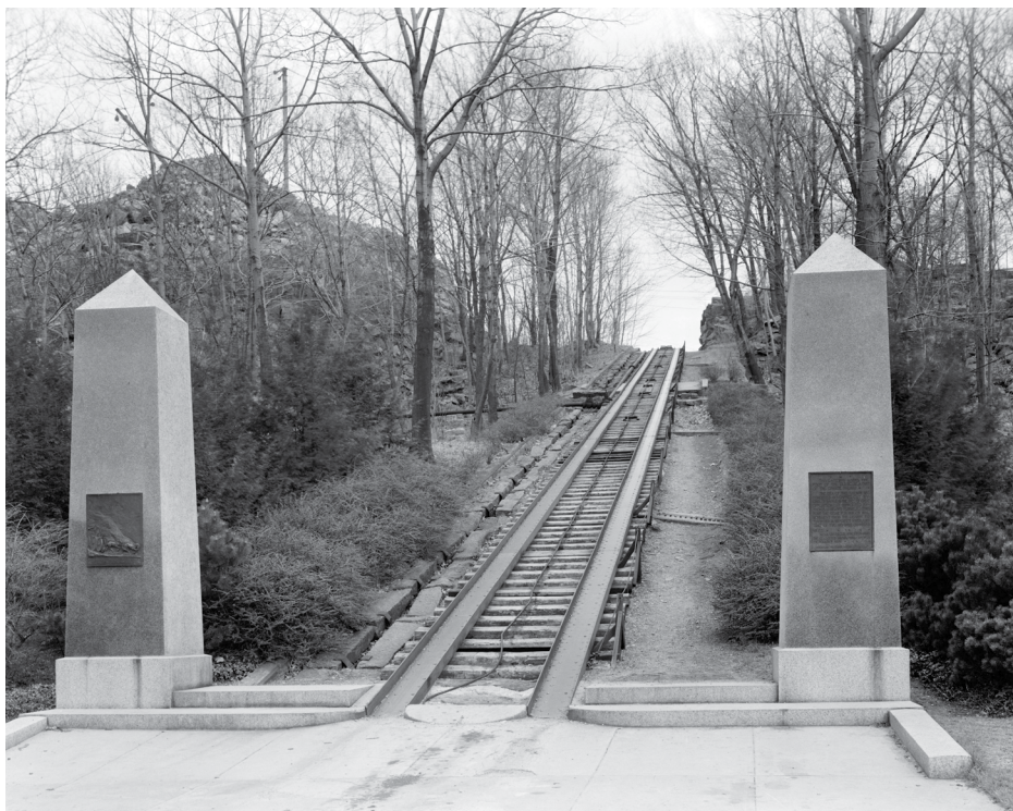
The Granite Railway, which opened in 1826, included this gravity-activated conveyor belt for bringing stone down from the quarry.
